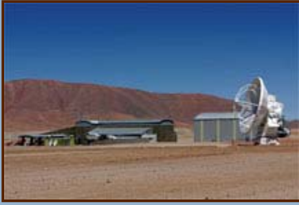
Fig. 1 The first ALMA antenna at the 5050m altitude Llano Chajnantor stands on pad 106. To its left is the Array Operations Site Technical Building that houses the correlator, the central local oscillator, and other equipment beneath the site's spectacularly clear skies. The antenna is controlled entirely from the lower elevation Operations Support Facility, a few dozen kilometers away.
