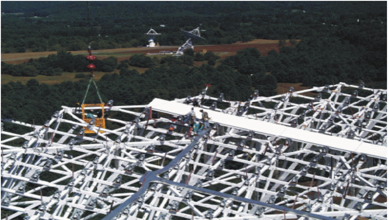
Completing the installation of the first tier of panels.
