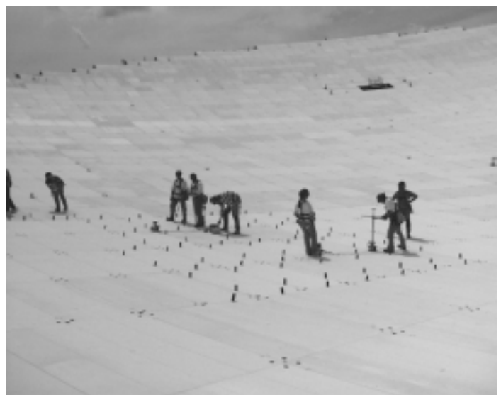
Setting surface-panel corners on the GBT.
